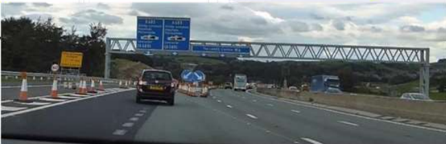
Super span gantry
